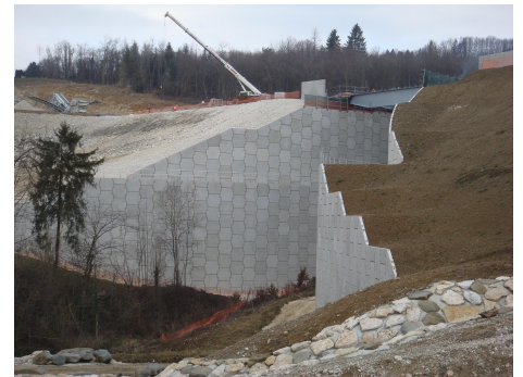
A41 Motorway - Bridge Abutments - La Ravoire - France
