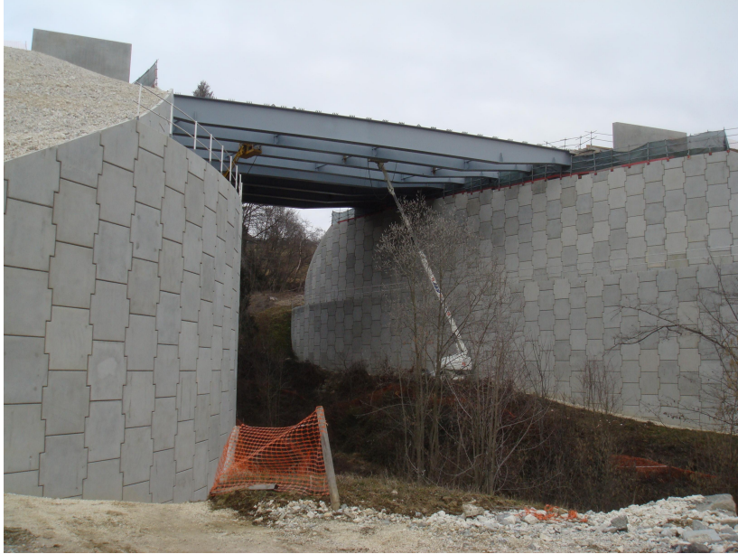
A41 Motorway - Bridge Abutments - Underpass/PI 161- La Ravoire - France
